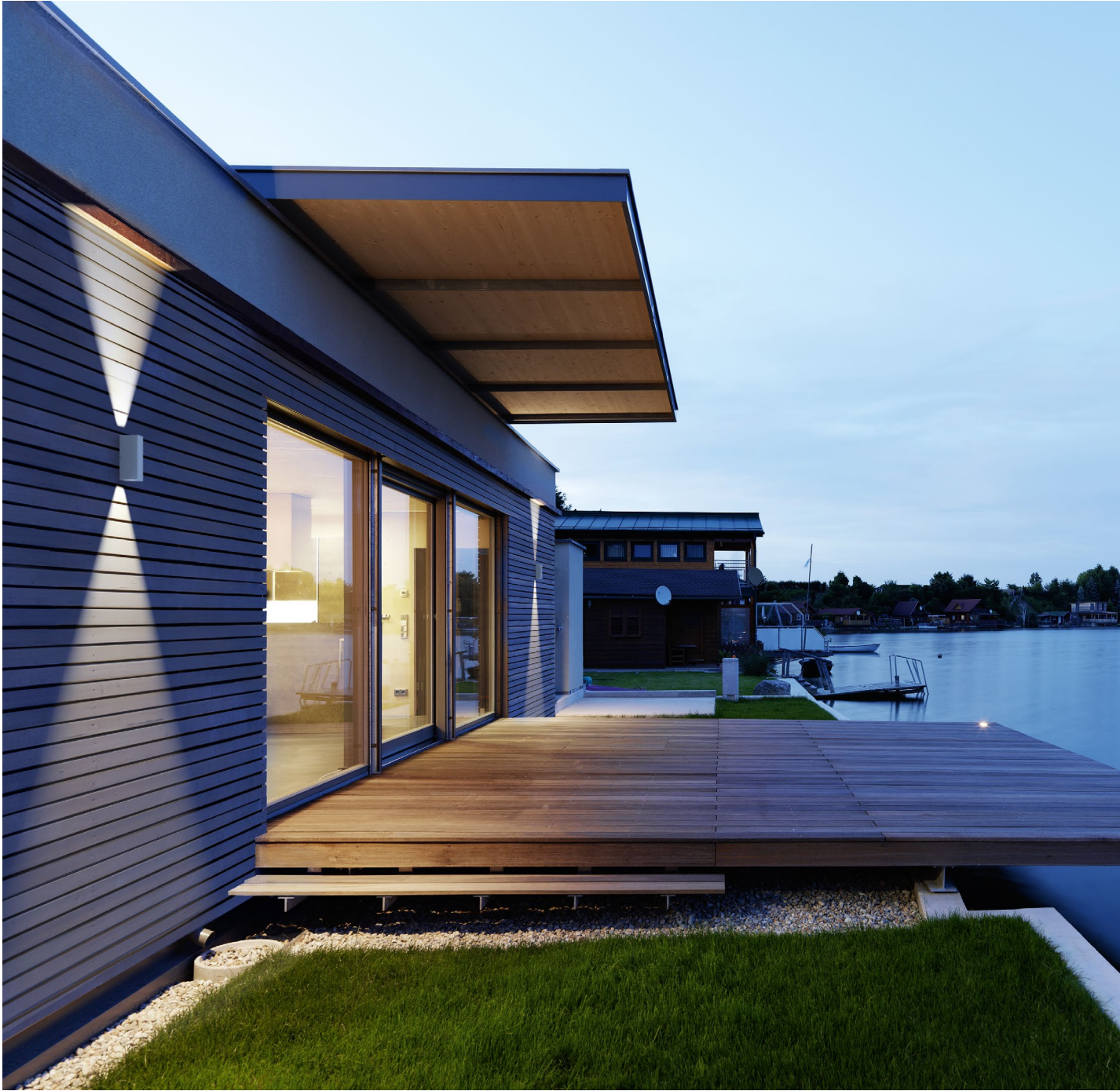
PRIVATE RESIDENCE | MOVING HOUSE | PILZARCHITEKTUR AUSTRIA
